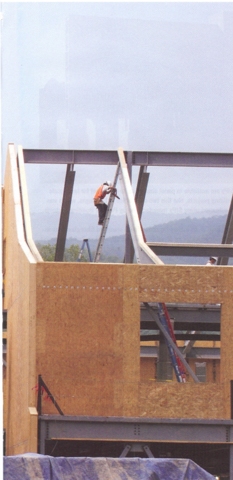
PHOTO: AL COBB, PANELWRIGHTS
