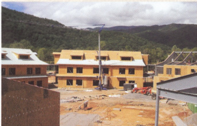
PHOTO: AL COBB, PANELWRIGHTS
